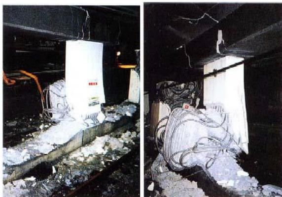
Fig. 2. Failure of central columns in Daikai station (Sato Industrial Inc. 1997)
