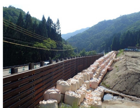
図-2.5.8 仮設防護柵
