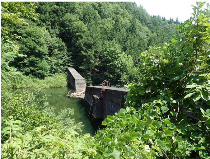
図-2.4.4 洞山谷砂防堰堤①
